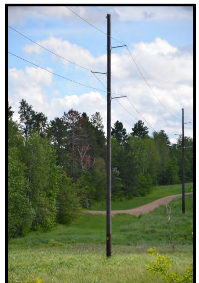
Typical 115 kV Wood Transmission Line Structure
